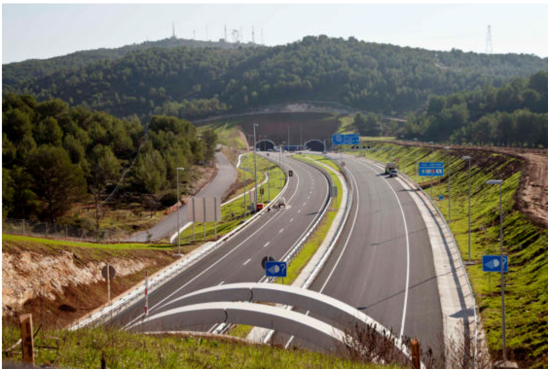
Túnel artificial Costa Bernada
